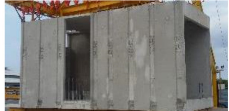
Reinforced concrete PPVC module
