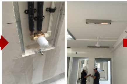
Weep Hole @ Toilet Recess and Electrical Final Fixing
