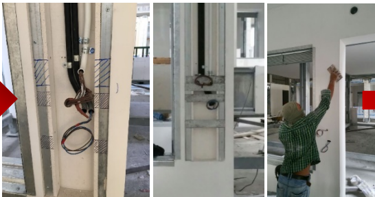
Electrical Work at Recess, Supporting Plate and Sealing Up
