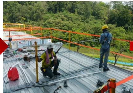
Waterproofing Sealant at Roof of PPVC Modules
