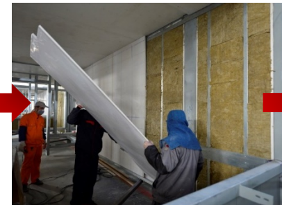
Rock Wool and Fire Board Installation
