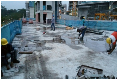
Setting up of final position of PPVC modules
