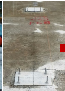
Setting up of final position of PPVC modules
