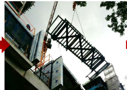
Installation of Link-way
