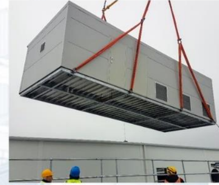
Level 4: MiMEP (in form of MiC) Free-standing integrated plant room module
