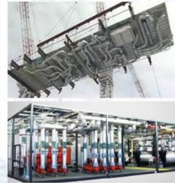
Level 3: MiMEP Multi-trade integrated unit; prefabricated plant room
