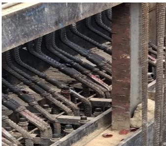
WK.LP Positional Coupler for Pile Cap Application
