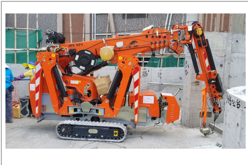
Photo : SPX424 at Lohas ph7 job-site
