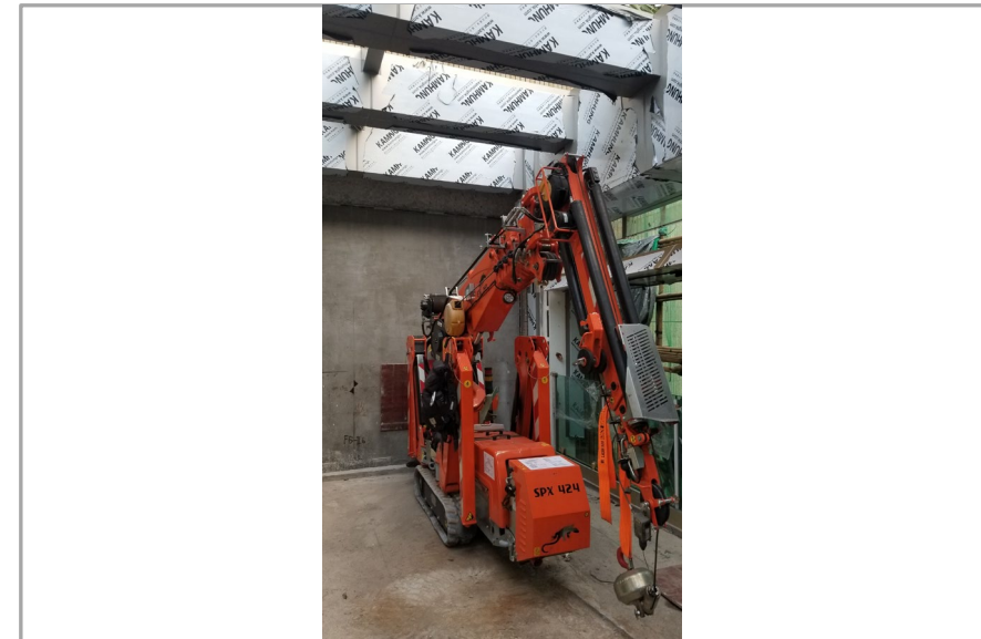
Photo : SPX424 at Lohas ph7 job-site
