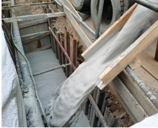
Filling with NAMI backfill materials
