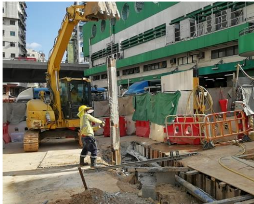
Removing sheet piles
