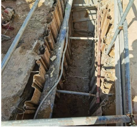
Trench before backfilling size: 4.0m*1.16m*2.3m
