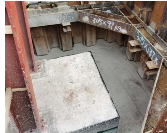
Excavation after backfilling
