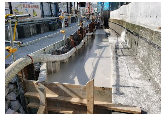
Excavation after backfilling
