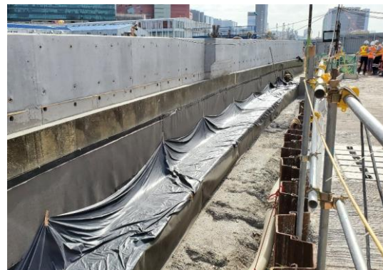
Excavation before backfilling
