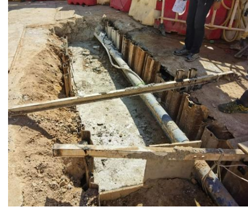
Trench after overnight
