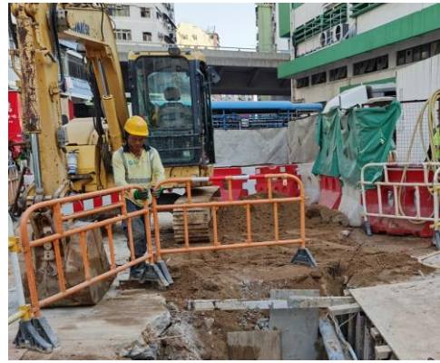
Filling the subbase
