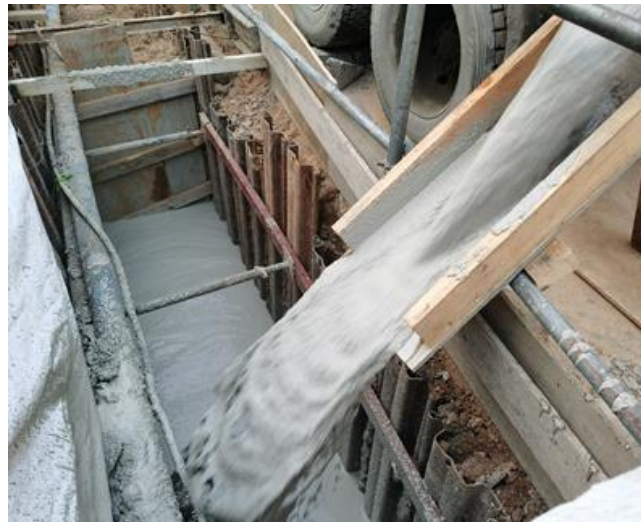
New method of backfilling by direct pouring of self-compacting backfill product
