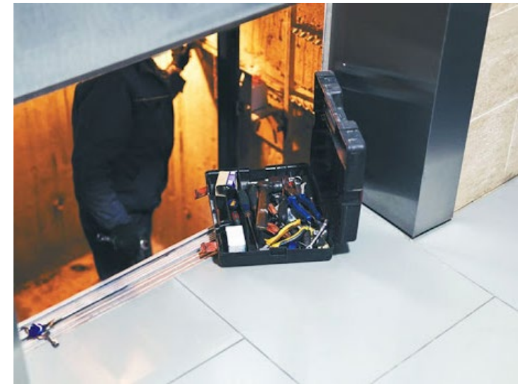
Traditional inspection – infrequent inspection can require early replacement of components
