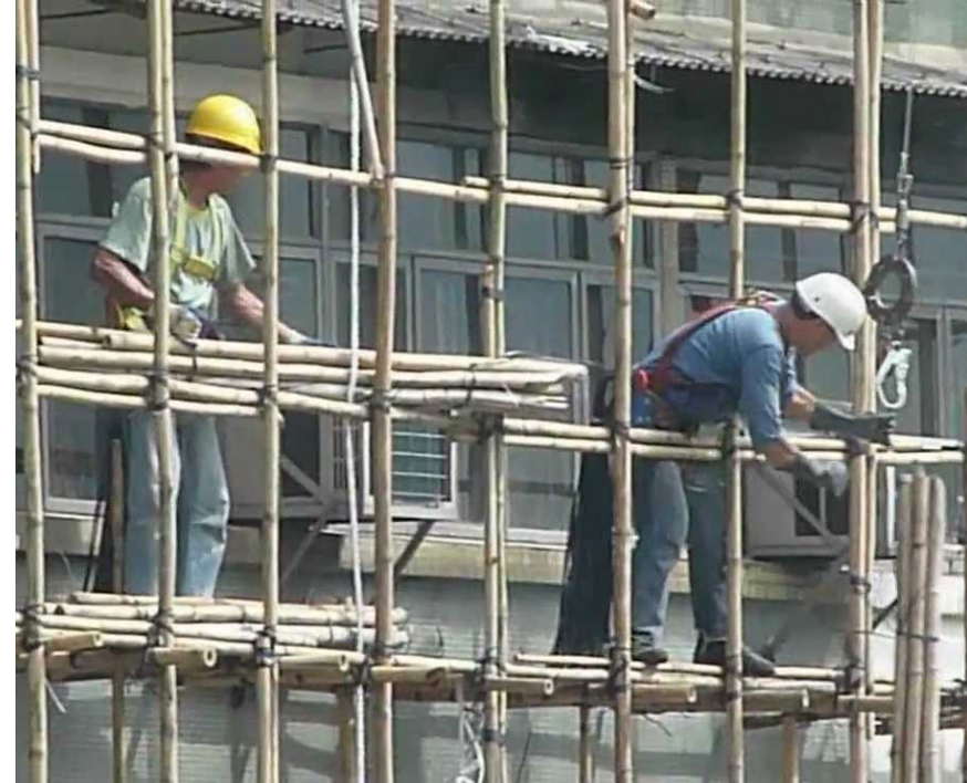
Manual scaffolding erection, as required in traditional inspection
