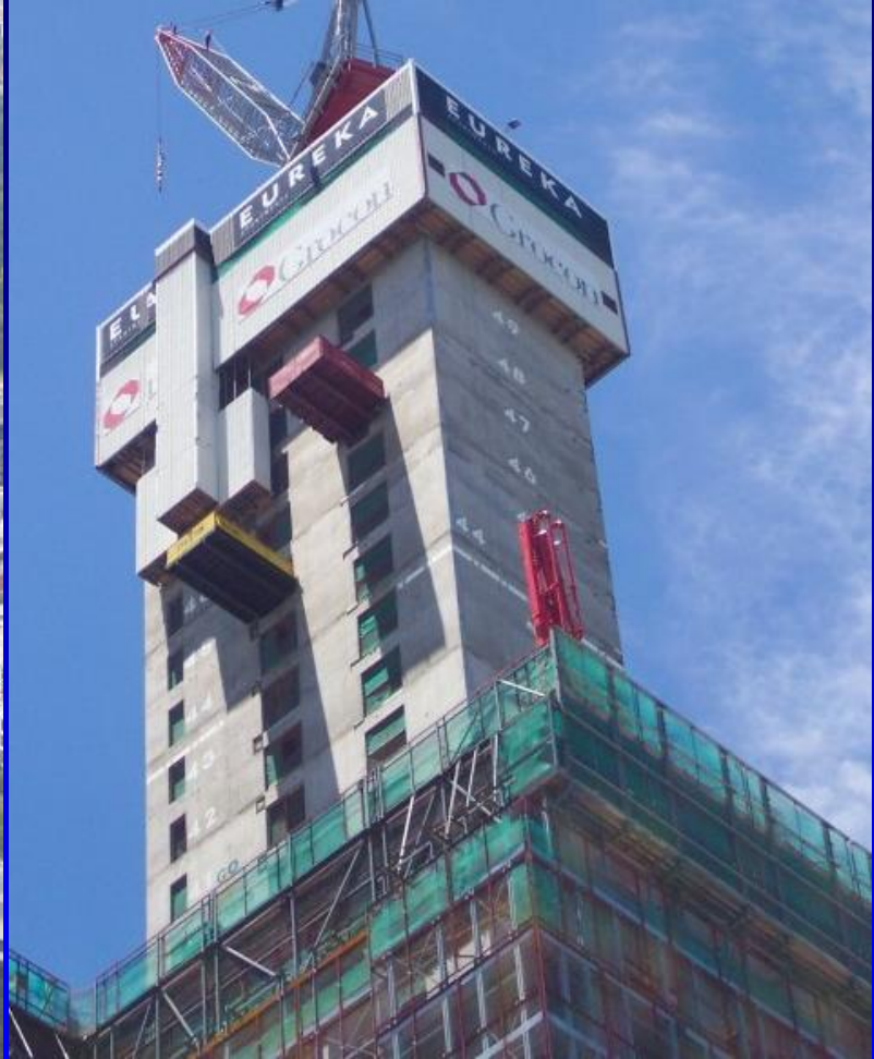
Typical example of an advanced formwork system-double storey jump (Eureka Tower Melbourne)
