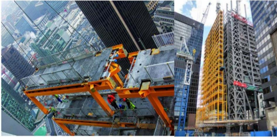
North Core and services integrated bench at The Leadenhall Building (Source: Davies 2013)
