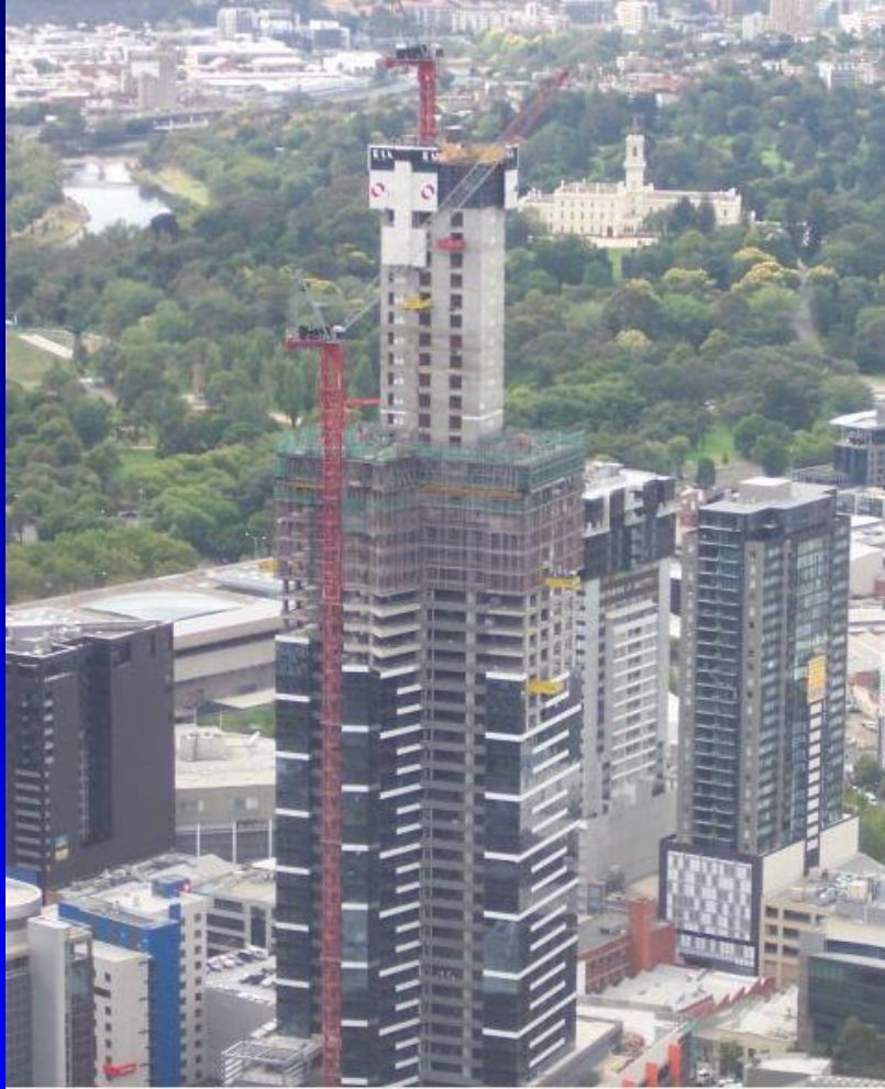
Typical example of an advanced formwork system-double storey jump (Eureka Tower Melbourne)
