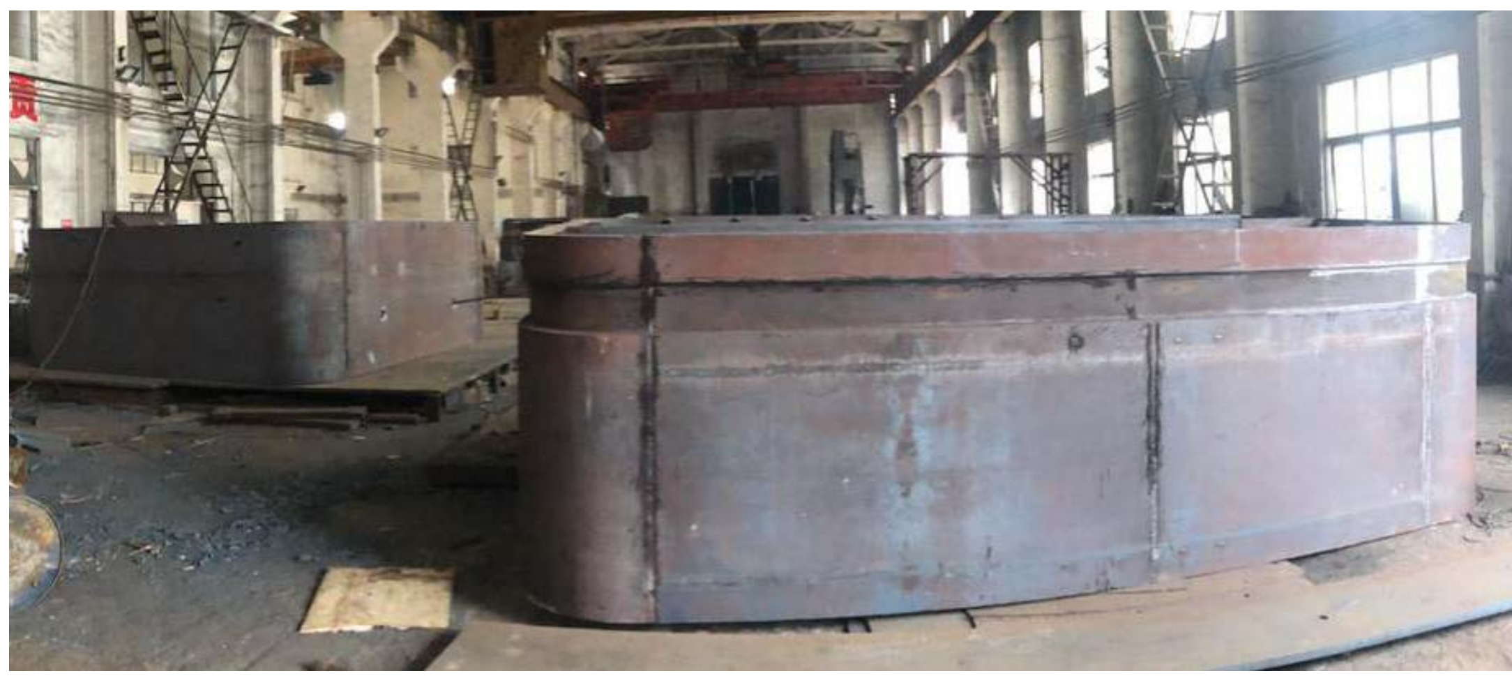
Front Shield body under Fabrication
