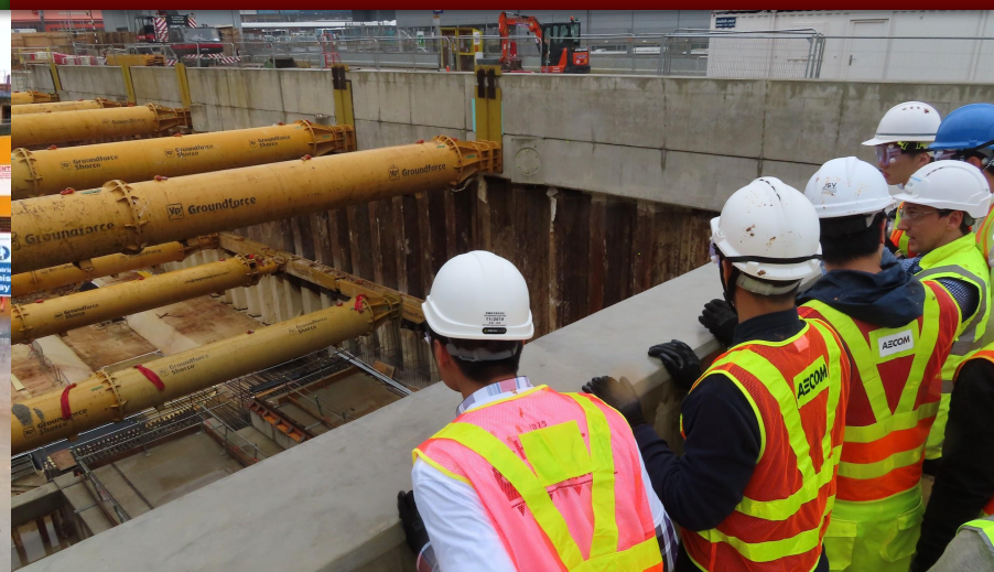
Excavation and Lateral Support (ELS)
