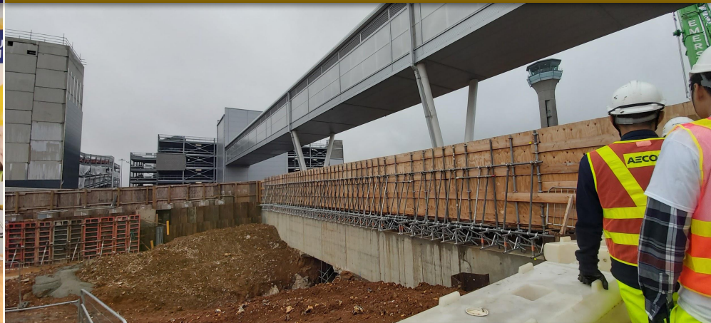
Excavation and Lateral Support (ELS)
