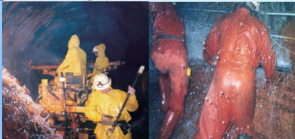
High Water Ingress During Tunnel Excavation
