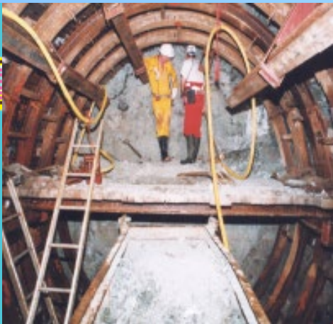
Pre-excitation Grouting & Manual Excavation
