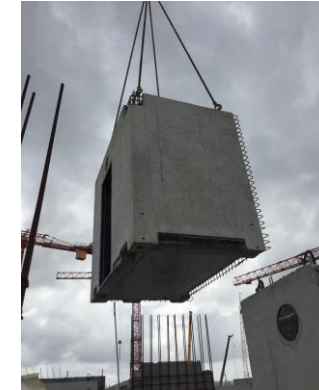
Load bearing precast wall and column, precast slab
