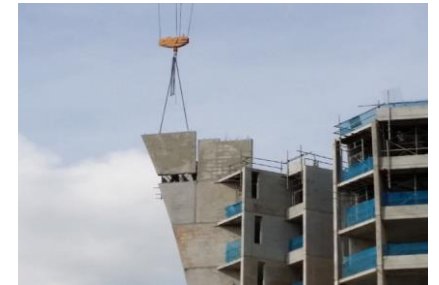
Load bearing precast wall and column, precast slab
