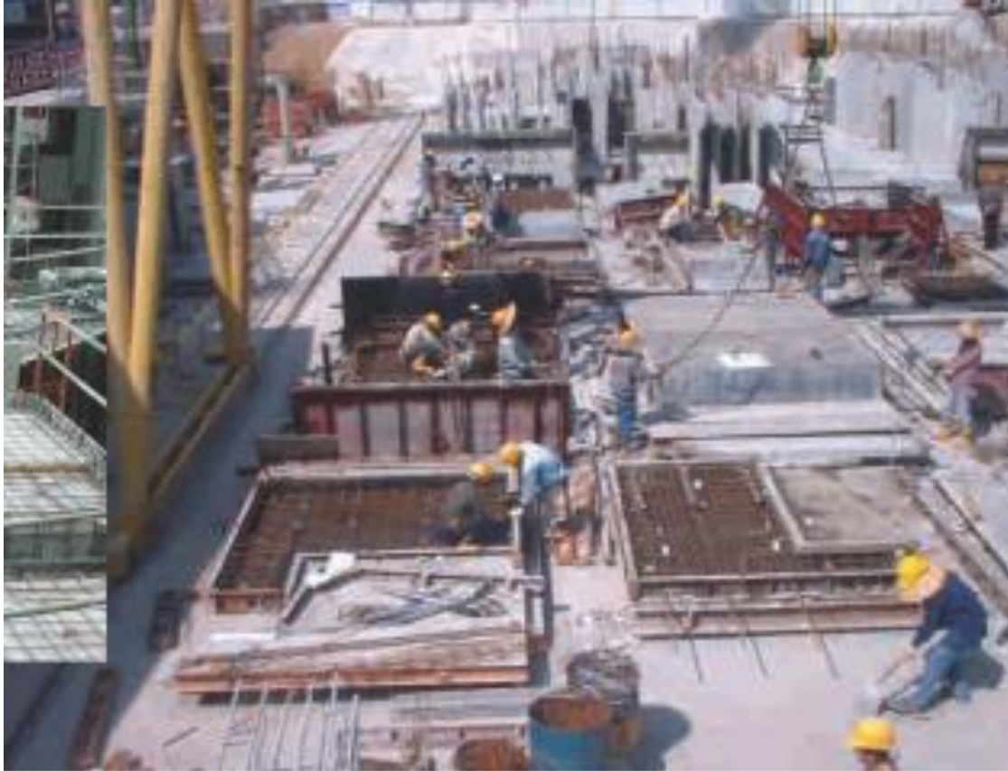
Fig. 6.11 – On-site precasting for simpler components
