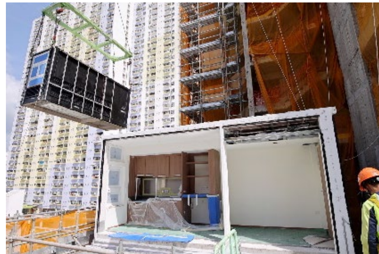
MiC module installation in progress
