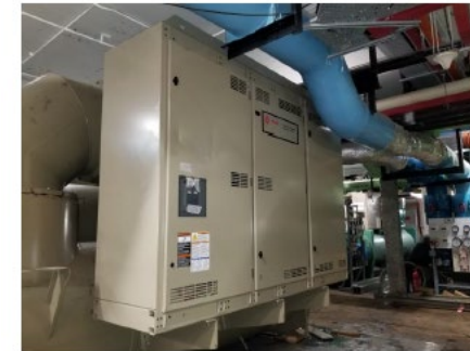
[Chiller and pipework setting out was reviewed by BIM]
