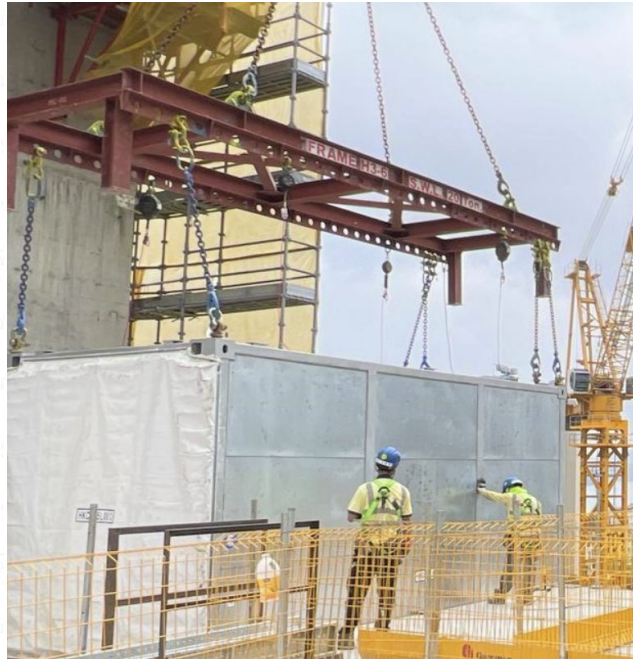
MiC module installation in progress
