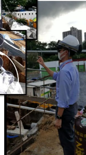
Trimble XR-10 download ifc Model Align in the Site
